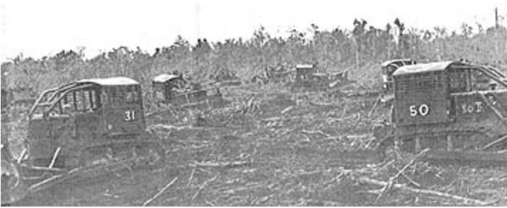
ROME PLOWS from the 60th Land Clearing Company clear the terrain and prepare a new night defensive position during the operation in the Crescent. (PHOTO BY SP5 DOUG ELLIOTT)
