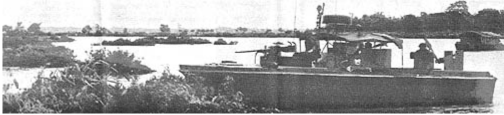
Equipped with five .50 caliber machineguns, this patrol boat searches the shoreline.
