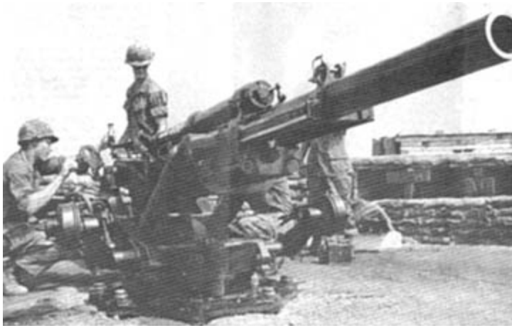
READY AND SET - Corporal Dale Dahlinger of Toms River, N.M., and Specialist 4 Doyle Reynolds of Bisbee, Ariz., assist in preparing the gun to fire. Dahlinger is setting the elevation of the tube while Reynolds rams the projectile into the breech. (PHOTO BY 1LT R.S. PERRY)
