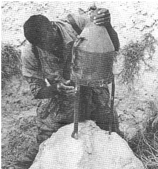
A 40-POUND SHAPED CHARGE will destroy the dirt mound used to support the heavy .51 caliber anti-aircraft guns. Specialist 4 Glen Davis of Kansas City, Mo., 65th Engineers, assigned to Company 3, 2d Battalion, 27th Infantry, skillfully prepares the explosive detonation. (PHOTO BY SP4 R.B. WILLIAMS)
