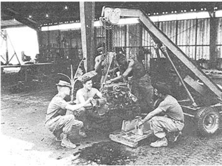
LIFT - An M-151A Engine is swung out onto a wooden frame for repairs.
