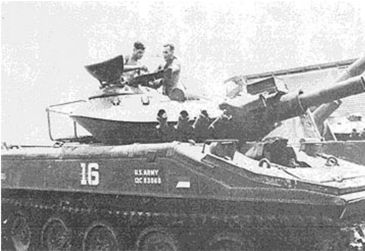
SHERIDAN - Among the routine adjustments the 725th makes are settings on the M88 pack of the new Sheridan tank.
