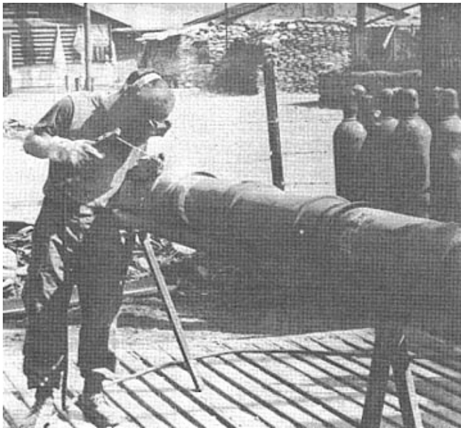
WELDING ARTILLERY propellant cans into 20-foot columns, a 'Triple Deuce' mechanic works to construct the 'Taj Mahal,' a giant all-weather maintenance facility. The welder is Private First Class Gerard Marceaux of Gueyden, La., a member of the battalion maintenance section.
