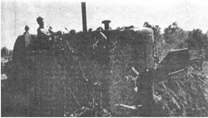
EARTH MOVER - Specialist 4 Leonard F. Cuprise of Degerton, Wisc, assigned to the 588th Engineer Battalion operates a D-7 bulldozer, clearing brush and forming berms at Tropic Lightning's Fire Support Base Stoneman, 15 miles southeast of Tay Ninh Base Camp.
