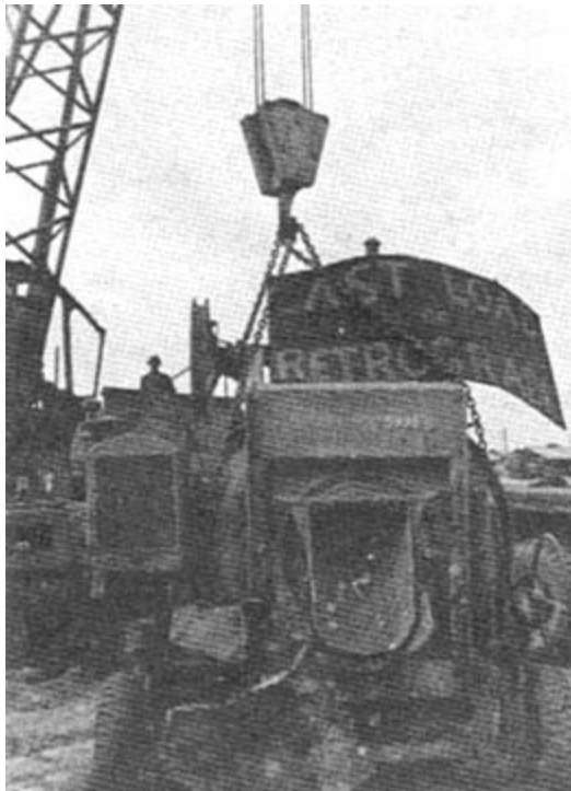
THIS CEMENT MIXER was the last load of retrograde to be removed from the Tay Ninh Retrograde Yard. In all, the 548th Maintenance Company of the 277th Supply and Service Battalion moved 4,507 tons of retrograde in five months from Tay Ninh to Long Binh (PHOTO BY 1LT MACK D GOODING)
