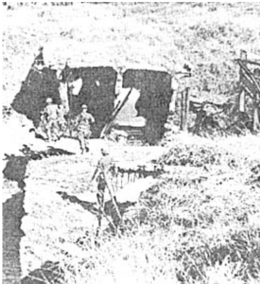
SECURING BRIDGE SITE - Men of C Company, 3d Battalion, 22d Infantry, move across the foundations of a demolished bridge on the Suoi Tri Bi River.
