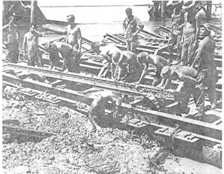
BRIDGE BUILDERS - Engineers of the 65th Engineer Battalion move a steel beam into place as they lay supporting members of the pontoon bridge. (PHOTO BY 1LT RICHARD SONSTELI)
