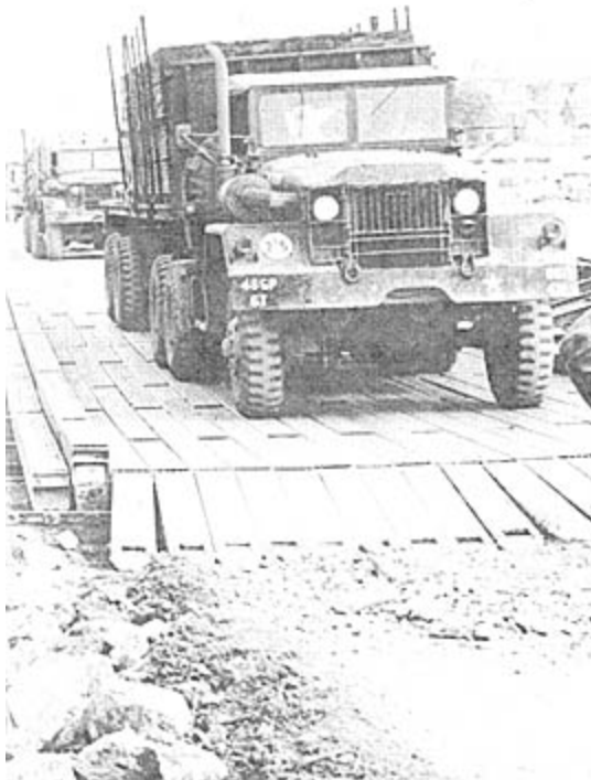
PONTOON BRIDGE - This pontoon bridge spanning the Saigon River was constructed through the joint efforts of U.S. and ARVN forces within 26 hours after the Phu Cuong bridge was damaged by enemy sabotage. (PHOTO BY 1LT J.N. BLACK)
