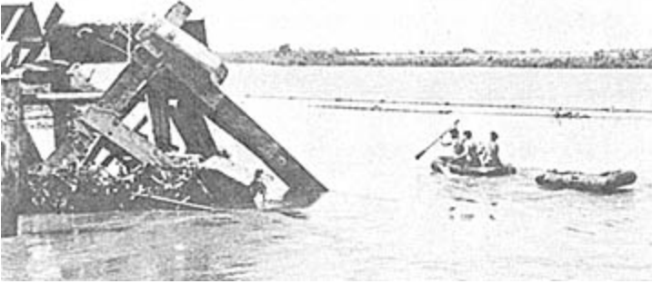
GREEN BERETS - Divers from Company A, 5th Special Forces Group, in Bien Hoa evaluate the DAMAGE TO THE Phu Cuong Bridge after enemy sabotage. (PHOTO BY 1LT J.N. BLACK)
