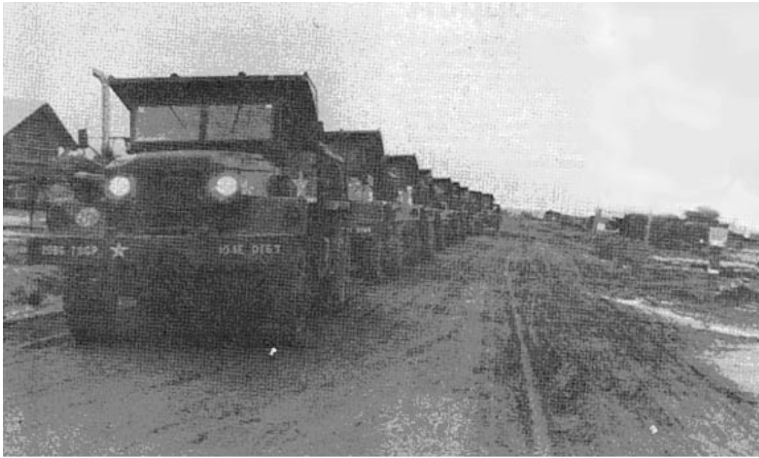
READY TO ROLL - Dump trucks from the 588th Engineer Battalion roll out of Tay Ninh carrying gravel for construction of a berm line at Bau Co. One hundred thirty-five trucks carrying seven tons of gravel each were needed to build the six-foot-high berm. (PHOTO BY SP5 RICK ADAMS)
