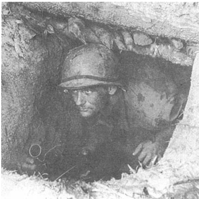
TUNNEL RAT - Specialist 4 Willie J. Sher of Indianapolis, Ind., inspects an enemy tunnel in the Iron Triangle. (PHOTO BY SP4 HECTOR NADAL)
