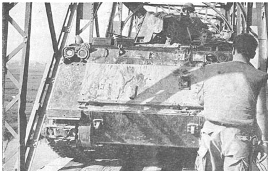
TIGHT SQUEEZE - APC's couldn't cross the Trang Bang River on the Eiffle-type bridge at the site; a new bridge had to be built.
