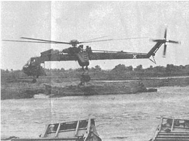
UP, UP AND AWAY - Everyone is across and the mission is complete as a CH-54 Skycrane removes the floats.
