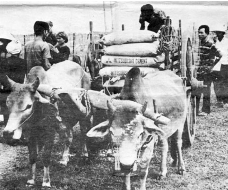
The people of Phouc Tan pick up the cement to begin the task of rebuilding.
